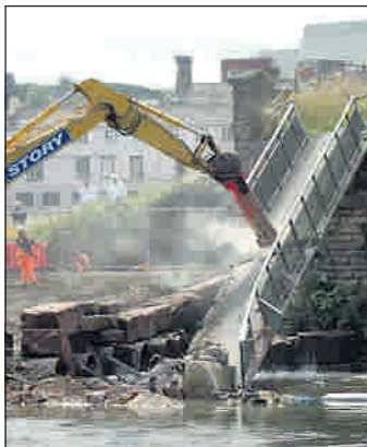
Demolished: Navvies Bridge has been cleared away
